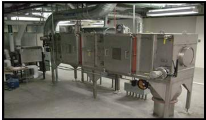
Figure 1-6. HEPA filtration plenum.
