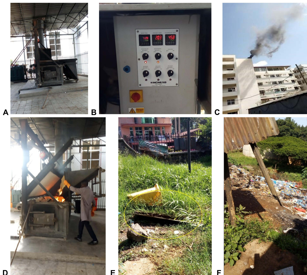
Figure 4 The photographs show the incinerator site (A), temperature display board (B), dense smoke emission from the chimney of the incinerator (C), fugitive emission and manual waste firing (D), placenta pit (E) and open dumping (F) in Jimma Medical Center, May, 2020.
